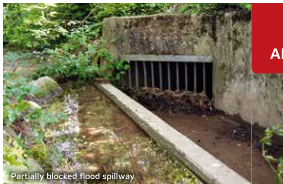
Partially blocked flood spillway
